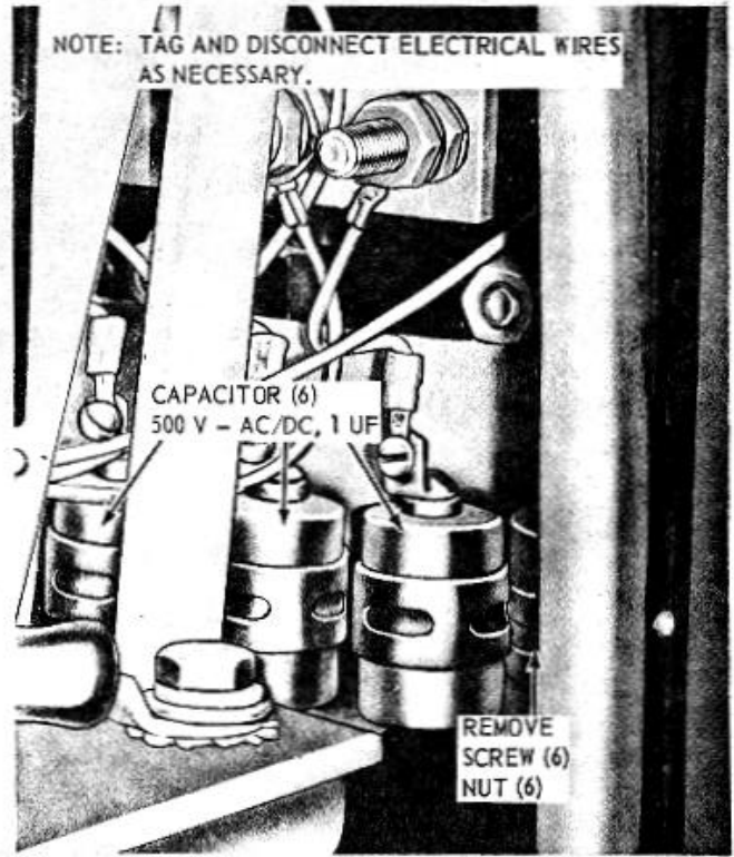
D. MAIN CIRCUIT BREAKER CAPACITORS.
